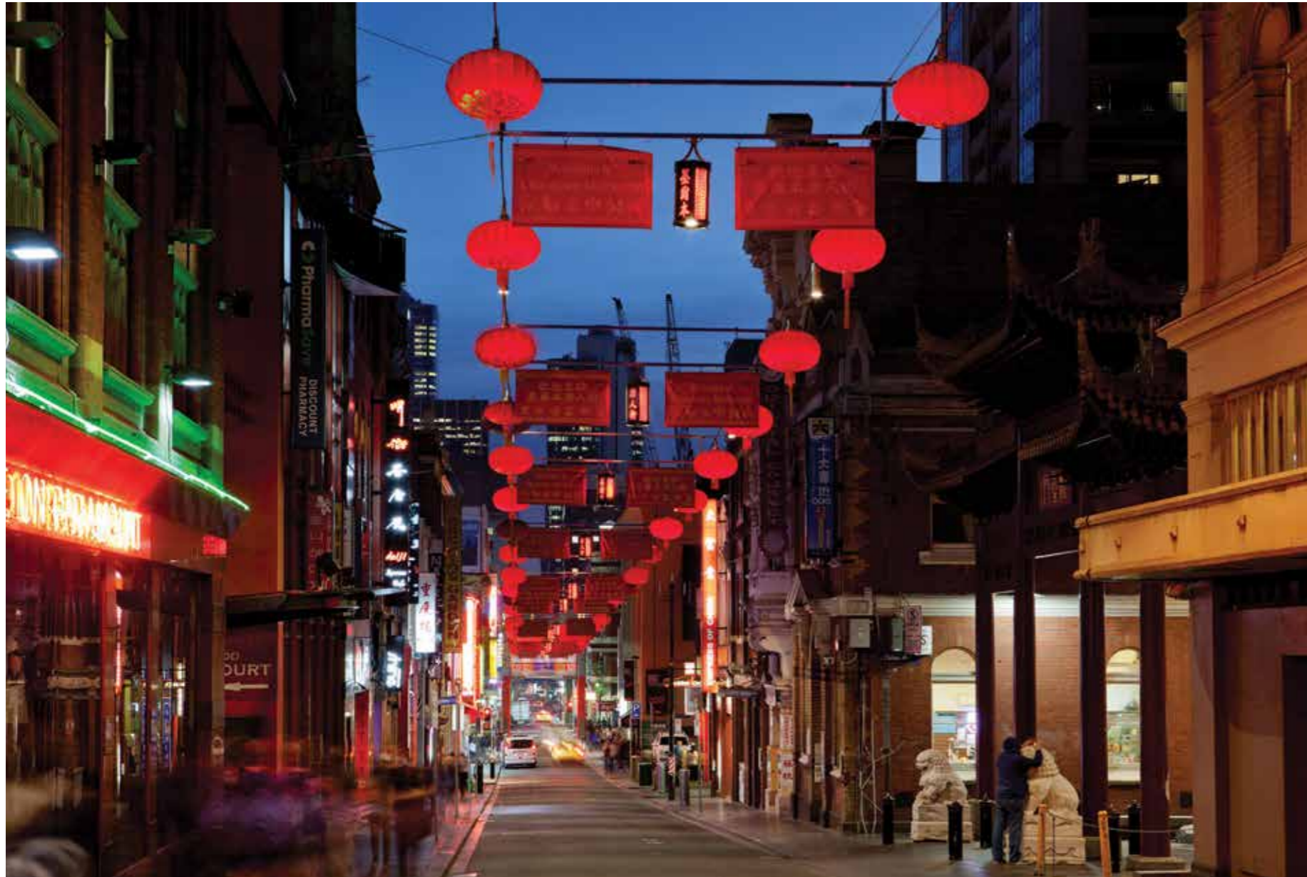
LED lighting installed in Melbourne's Chinatown Catenary.
