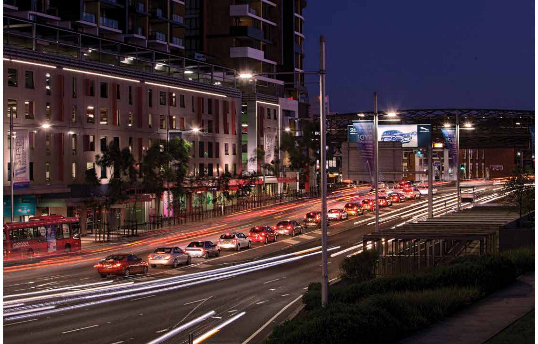
Smart arterial LEDs over Ryde Road in the City of Ryde.
